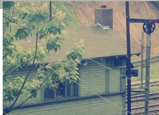
Above Photo: Vertical building corner L shape boards.
